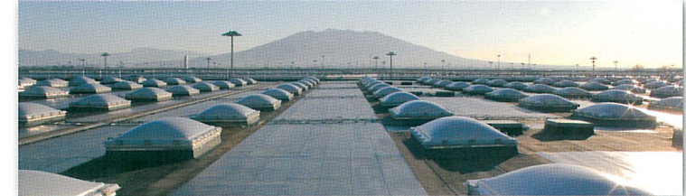
Stopping the Water and Catching the Sun in Nola (Naples) with the world's largest integrated roofing system for waterproofing and energy production. 25 MWp installed that will produce 33 million kWh (equivalent to 13.000 households).
