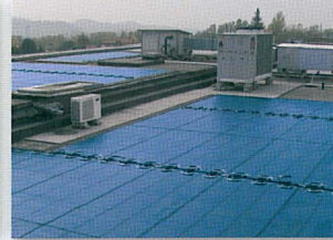
APPLICATION OF GENERAL SOLAR PV® ON THE EXISTING ROOF, WITHOUT DRILLING THE ROOF
