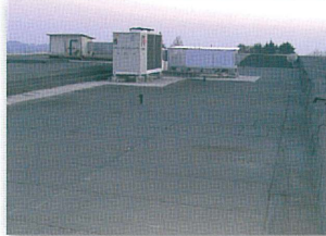
EXISTING ROOF WITH BITUMINOUS WATERPROOFING MINERAL MEMBRANE
